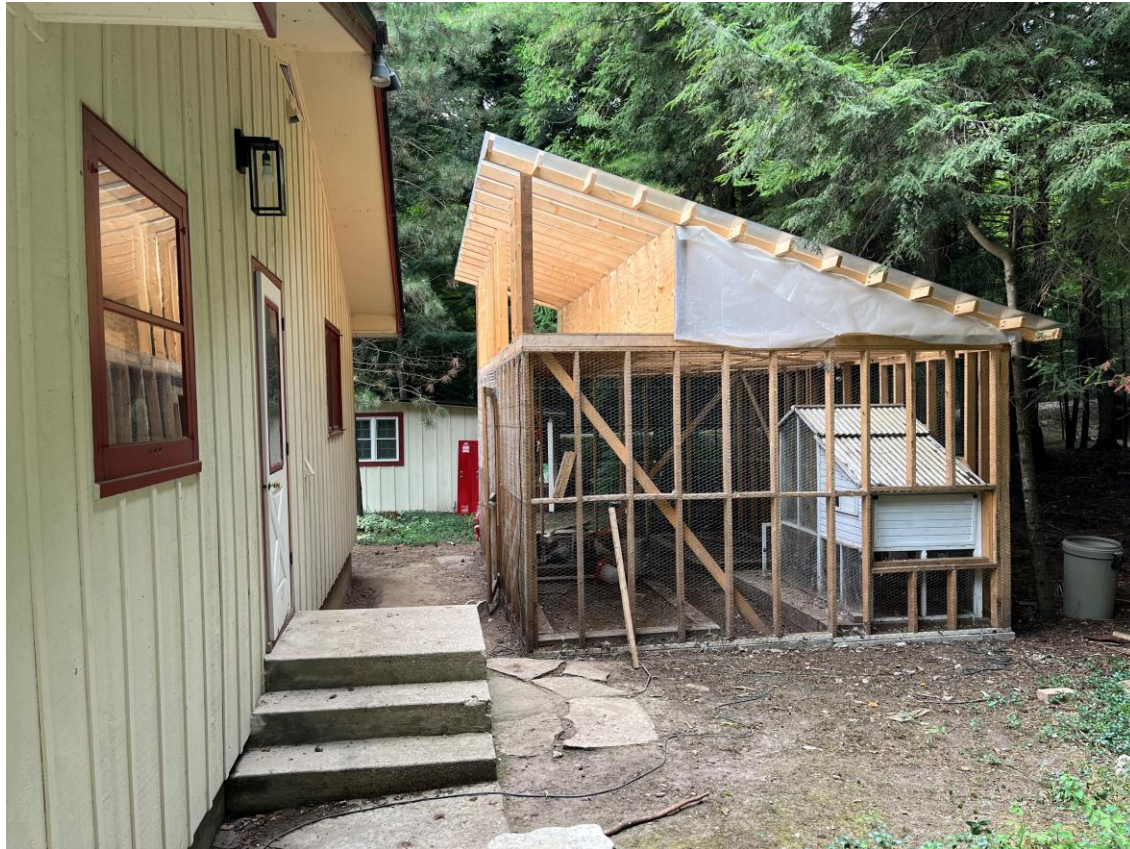
Structure as it is now
