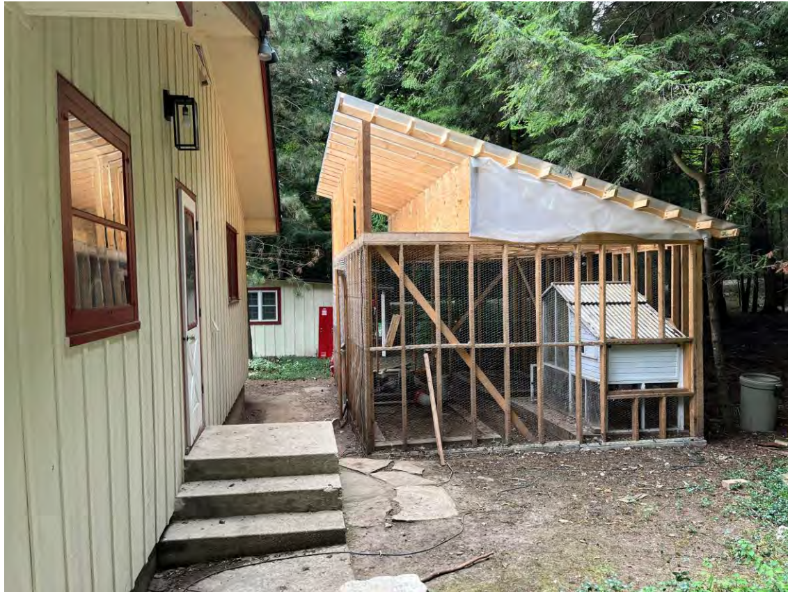
Structure as it is now
