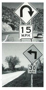
The advisory speed must be determined by an accepted traffic engineering procedure but no ordinance is required. Maintenance or sign supervisors can erect the signs. They must be in accordance with guidelines in the *MUTCD, 2C-35.*
